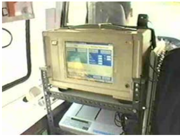
Figure 2. The interior of the ambulance before the installation of the new 12-lead ECG module.
